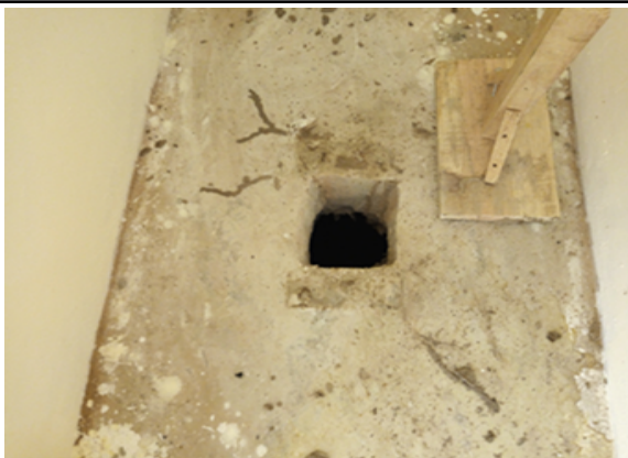
The inside of one of the Latrines without floor slopes
